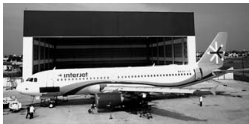
Interjet's maintenance base at Toluca Airport maximizes efficiency to cut costs and to attract foreign carriers.
