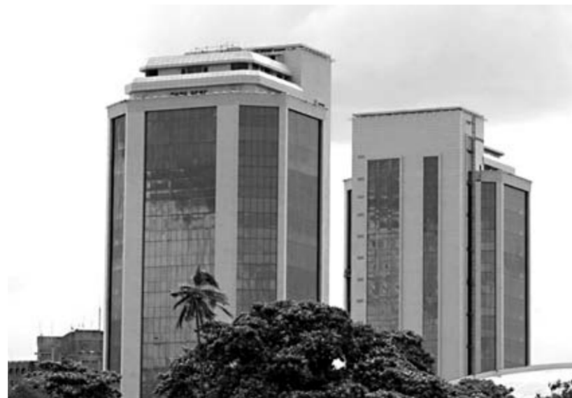
The loans that the Tanzanian government has received will go towards infrastructure and other social development projects to assure that the nation can continue on its path of steady growth
